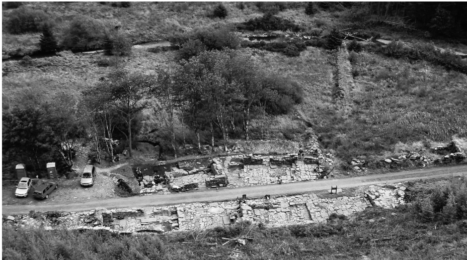
Figure 1: Excavation in progress on the manor house at Dolwyddelan, North Wales. (photograph by the author).
