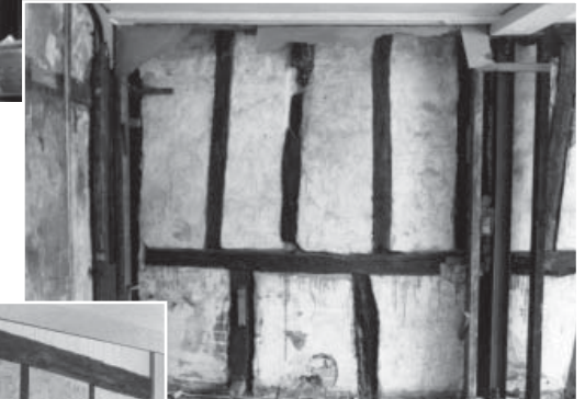
Figure 3 (below): Murals during demolition work.
