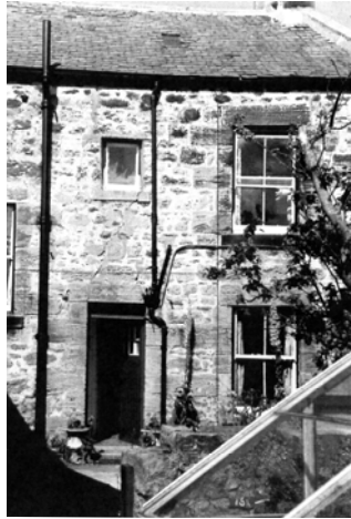
Figure 7: Rear of 13 Yard Heads, photograph taken 1980s.
